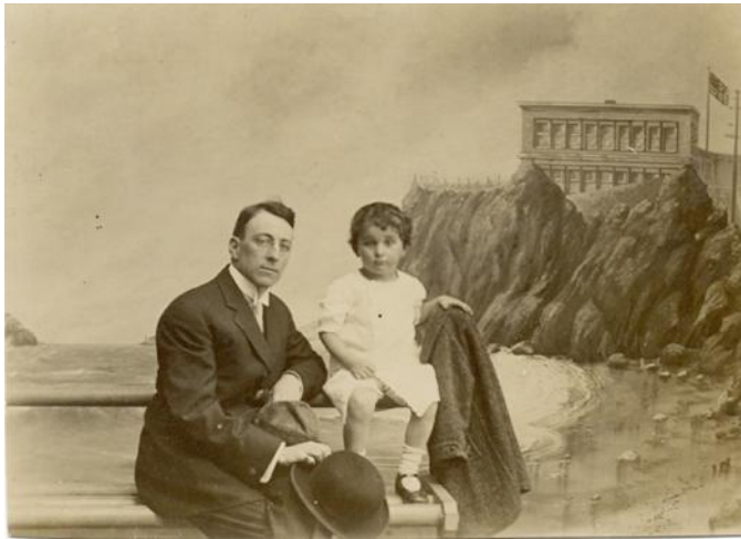
Above Jack with son at Cliff House, San Francisco, 1910
